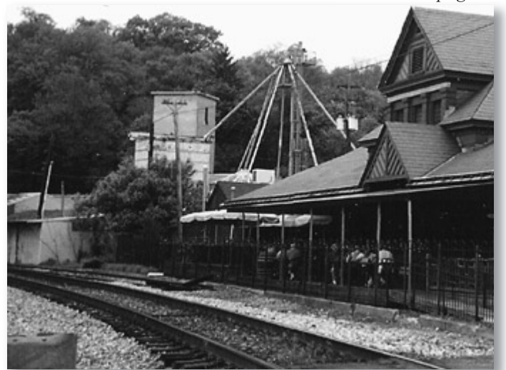
Baldwin's Station today.
